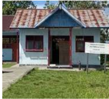
Figure 1. Public Elementary School 5 Kampung Puay
